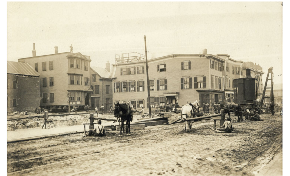
Dor. Tun. Sec. J, Moving "3-Flatter" along Dexter St. looking NW'ly. June 7, 1916. #1153-D
