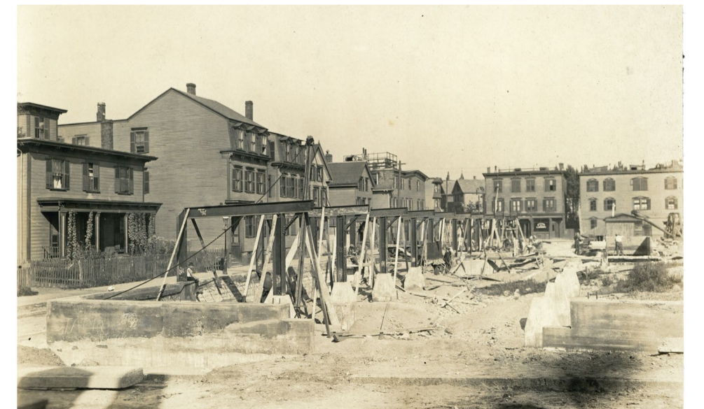
Dor. Tun. Sec. J, Andrew Surface Station. Erecting Steel. Sept. 13, 1917. #1534-D
